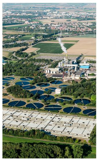
The BASF wastewater treatment plant at the Ludwigshafen site in Germany is one of the largest in Europe. Around 86 million cubic meters of production wastewater are treated here every year, plus around 18 million cubic meters of wastewater from surrounding communities. In recent years, we have continuously increased ne energy efficiency and effectiveness of the plant.
